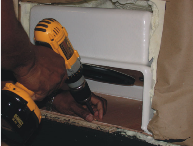
Figure 13. Attaching to Frame
